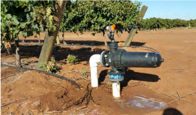
AUSTRALIA AUSTRALIA | Irrigation Riego
