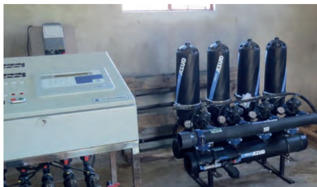
ZAMBIA ZAMBIA | Irrigation Riego
